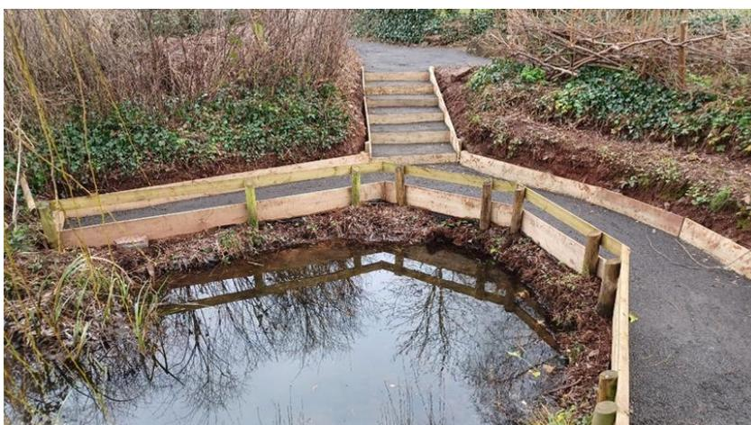
water level. To make it easier and safer, we engaged an excavator contractor to dig down the standing level by 30cm. The Canal Rangers and volunteers then edged the paths, built new steps and used crushed stone to re-surface all around, including the main path through the garden which had been becoming increasingly puddy.
